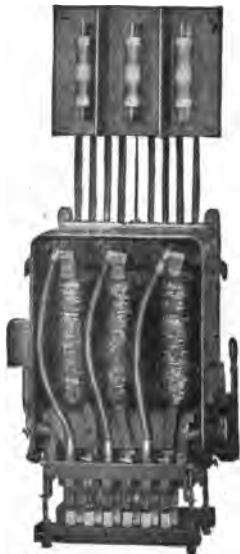
FIG. 251. Three-phase starting compensator for induction motors, equipped with no-voltage release (left side) and fuses to protect against overload. The cylinder switch at the bottom is for making the starting and the running connection.
